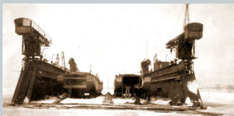
Two MFP on repair in the dock of Varna. Photo: Collection Reinhard Kramer.
